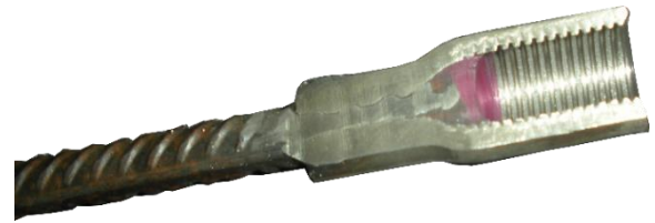
The illustration shows a sliced transport anchor with this seal.
