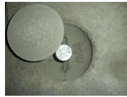
**BGW sealing plug made of glass fibre reinforced concrete Distance holders, Sealing cones, exposed concrete cones**
